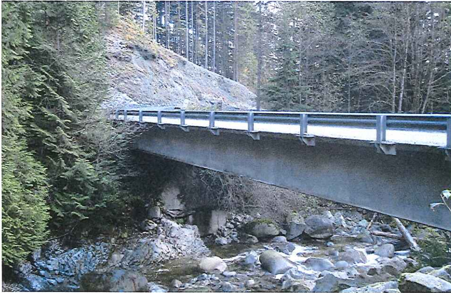
CK-2093 Crossing Upstream
