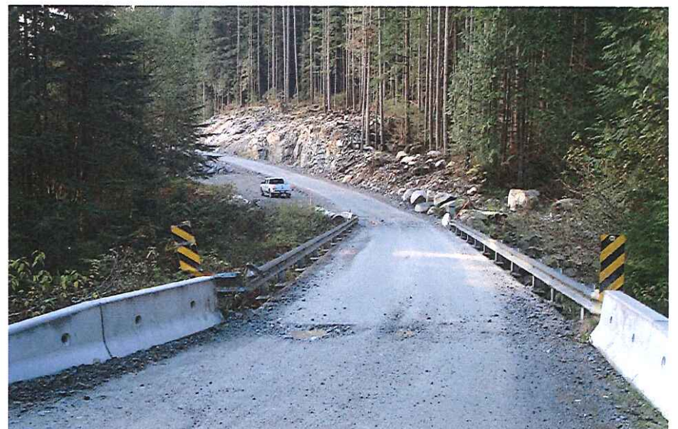
CK-2093 Approach Left Bank
