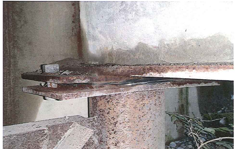
CK-2093 Condition of Bearing Pads
