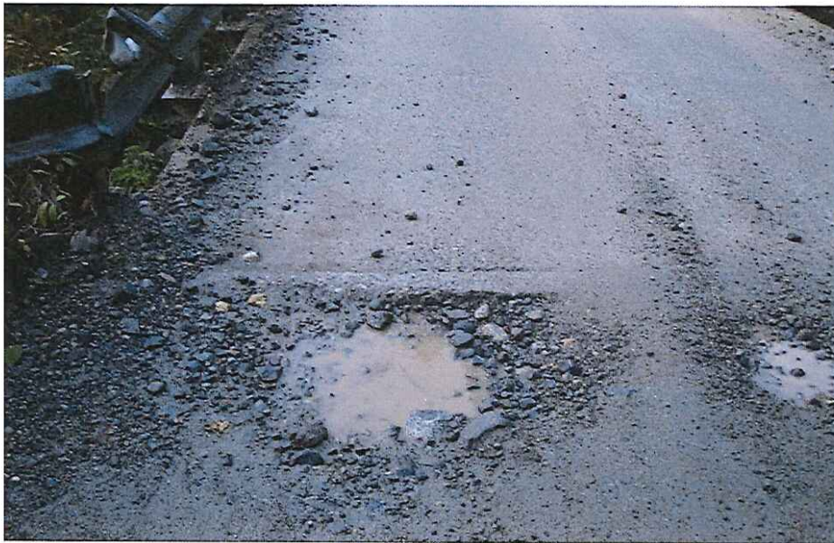
CK-2093 Condition of Approaches
