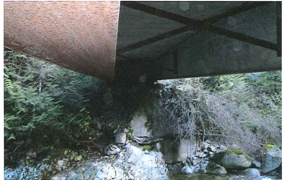
CK-2093 Abutment Left Bank
