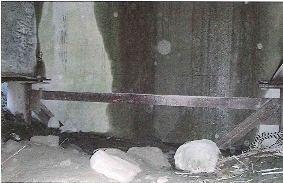
CK-2093 Abutment Right Bank
