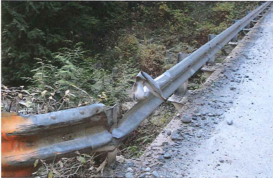
CK-2093 Downstream Left Bank Guardrail
